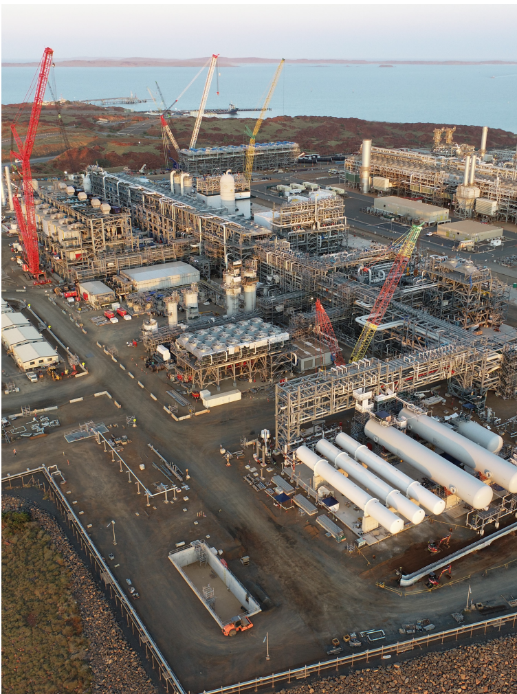
Figure 1 – Pluto Train 2 site
