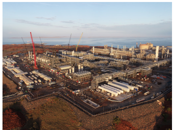
Pluto Train 2 construction progress, Western Australia, December 2024
