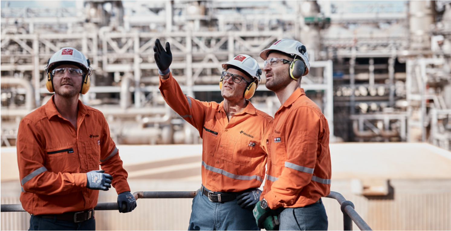
The Karratha Gas Plant in Western Australia has been providing a reliable and affordable supply of natural gas to domestic and international customers for decades
