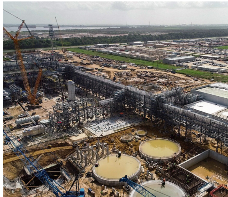
Construction of the Beaumont New Ammonia Project, July 2024
