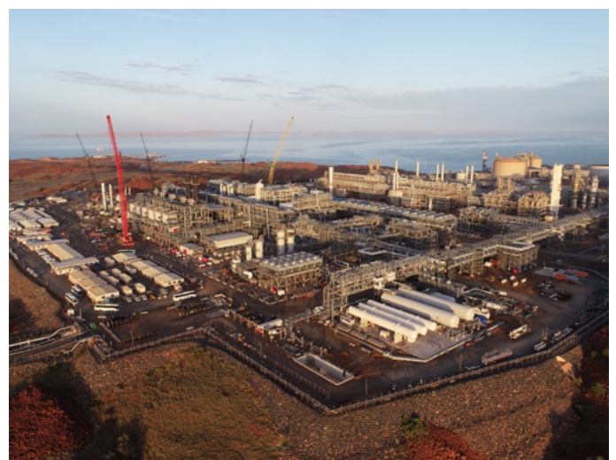
Pluto Train 2 construction progress, Western Australia, December 2024
