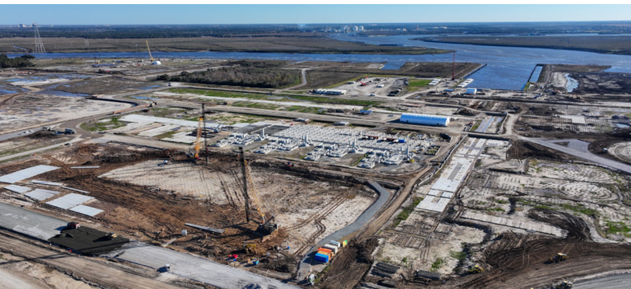
Woodside Louisiana LNG development, January 2025
