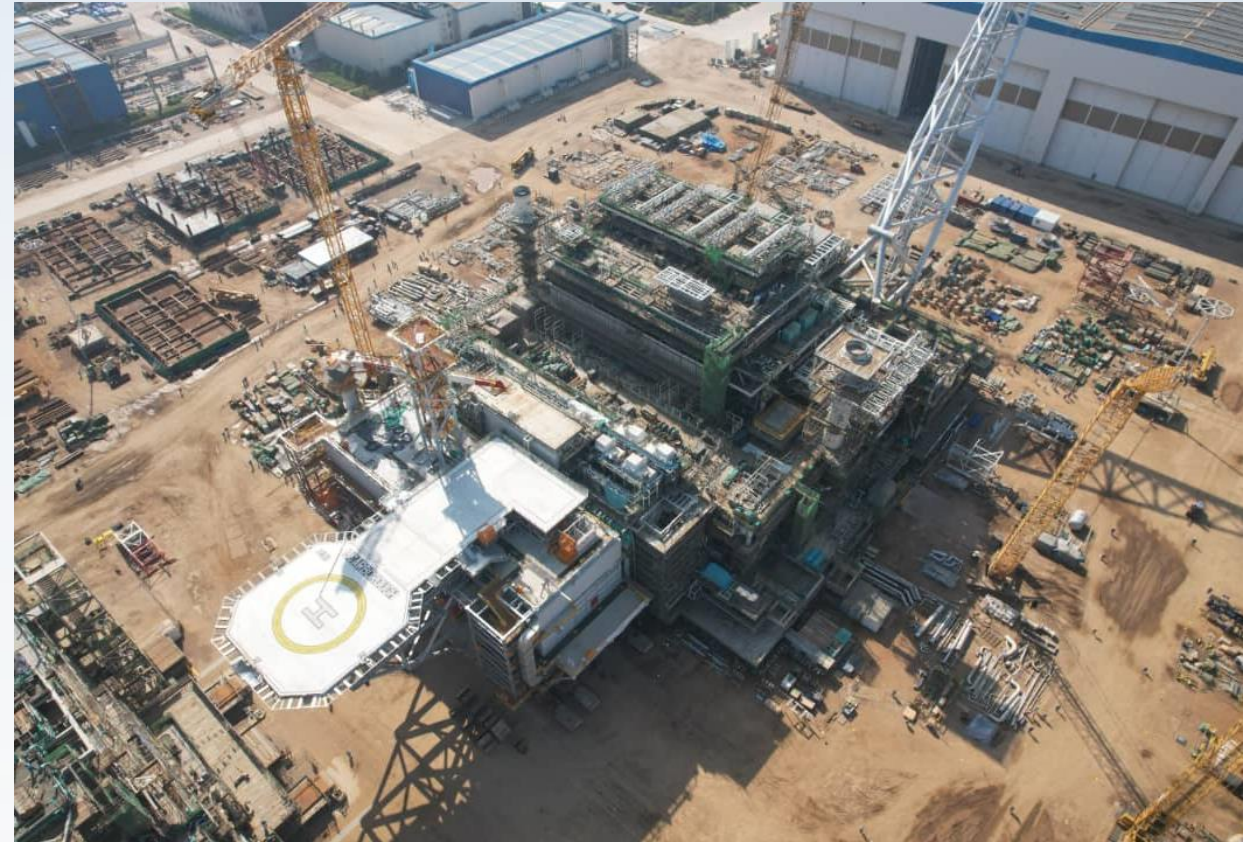
FPU topsides construction
