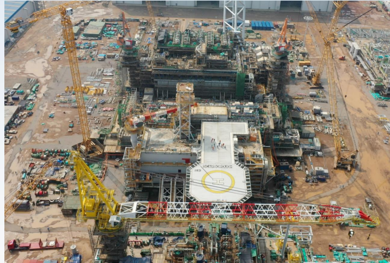
Floating production unit topsides progress
