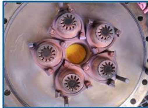
Methane: GTG nozzles replacement
